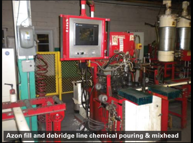
Azon fill and debridge line chemical pouring and mixhead exit side
